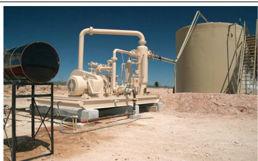
Vapor recovery units can recover more than 95 percent of the emissions that accumulate in crude oil storage tanks. The gas makeup of the vapors varies, but methane generally accounts for 40-60 percent of the total gas stream. Also, since the recovered vapors contain liquids, the Btu content is much higher than pipeline gas, making the recovered vapors more valuable than methane alone.
